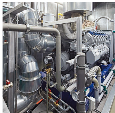
MTU's upgraded BHKW 2.0 runs on biomethane and, compared to conventional co-generation plants, generates power much more efficiently and cleanly.
